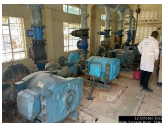
Photo 2-1 Raw / Treated water pumping station house and WTP dosing plant
